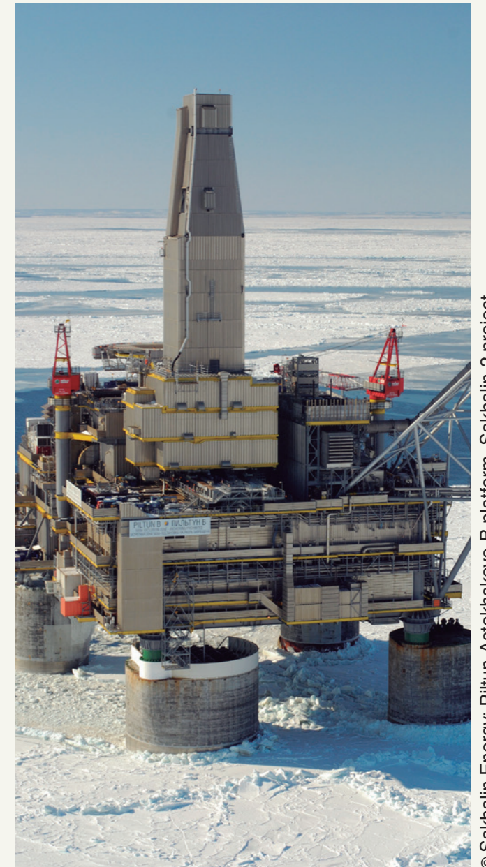
© Sakhalin Energy: Piltun-Astokskoye-B platform, Sakhalin-2 project.
